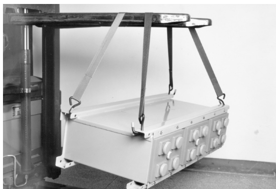
Figure 5: Positioning the module onto the base channels
